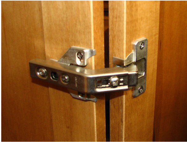
Figure 3: Blum Bi-fold Hinge Configuration
